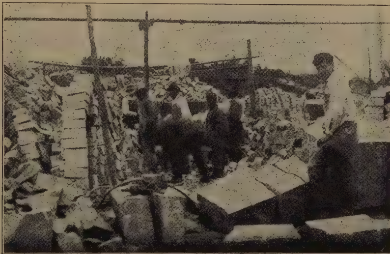
Piles of Finished Paving Blocks. Compressed Air Drilling Machine Resting on Bigger Blocks.—From Lohrville, Wis.
